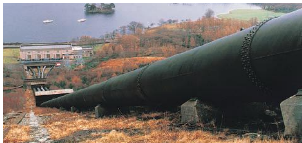
d Potential energy of water to kinetic energy of turbine to electrical energy from generator
