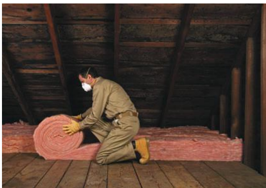
Figure 23.4b Laying lagging in a house loft
