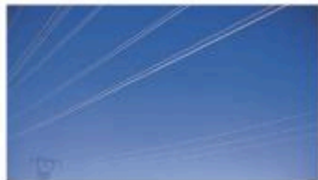
Figure 17.12 Aluminium resists corrosion, has a low density and is a good conductor of electricity – the aluminium in the cables is strengthened by a core of steel.
