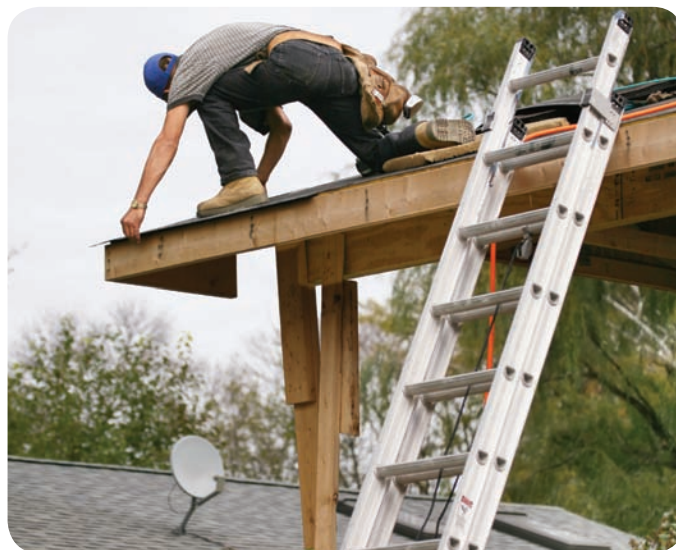
▼ The aluminium ladder is protected from corrosion by its oxide layer.
