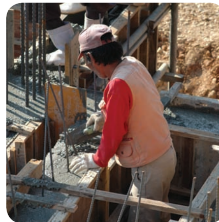
▲ Cement: limestone heated with clay – and gypsum is added to slow down the 'setting' process.
